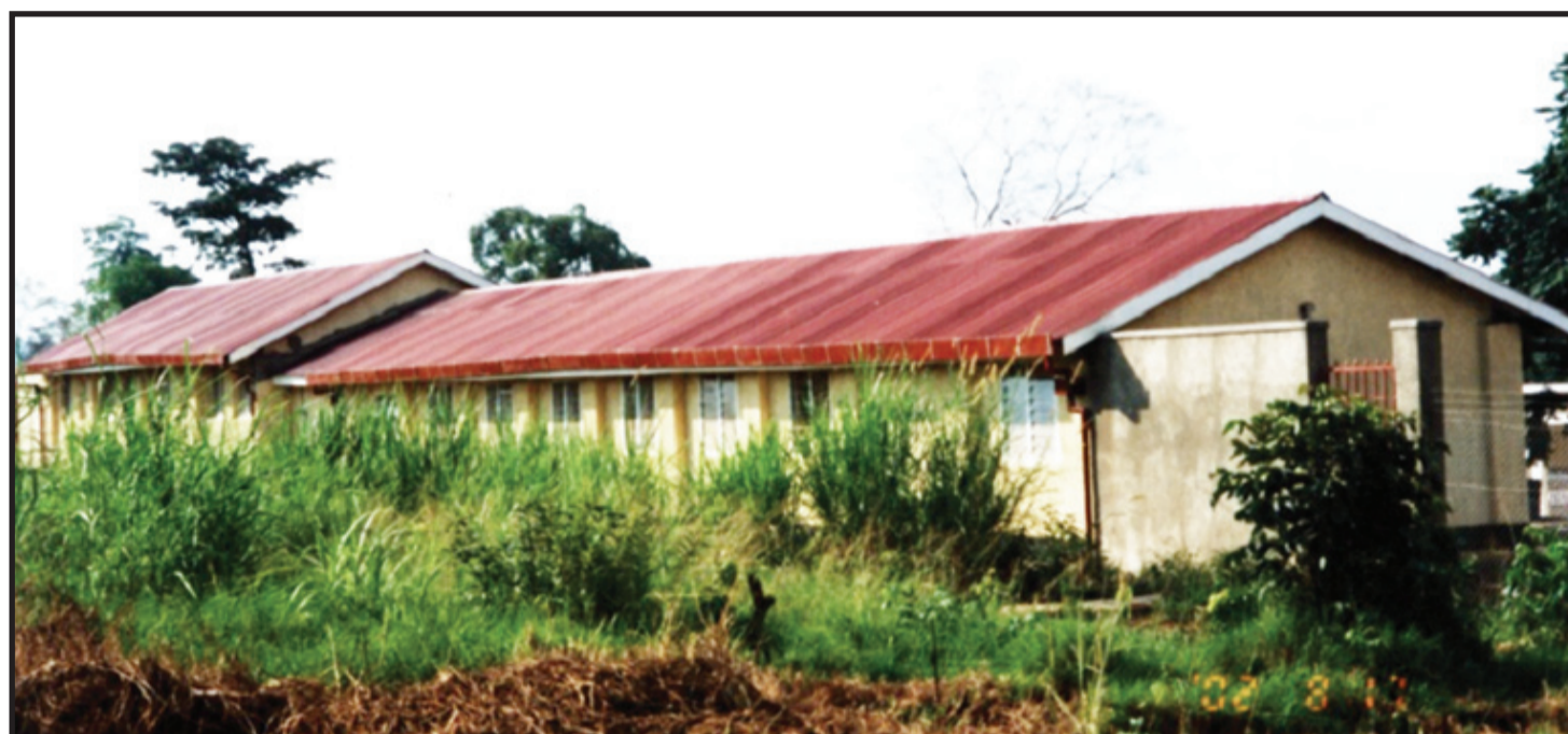
Former Kitemba Primary School which currently houses offices for Kaweeri Coffee plantation
