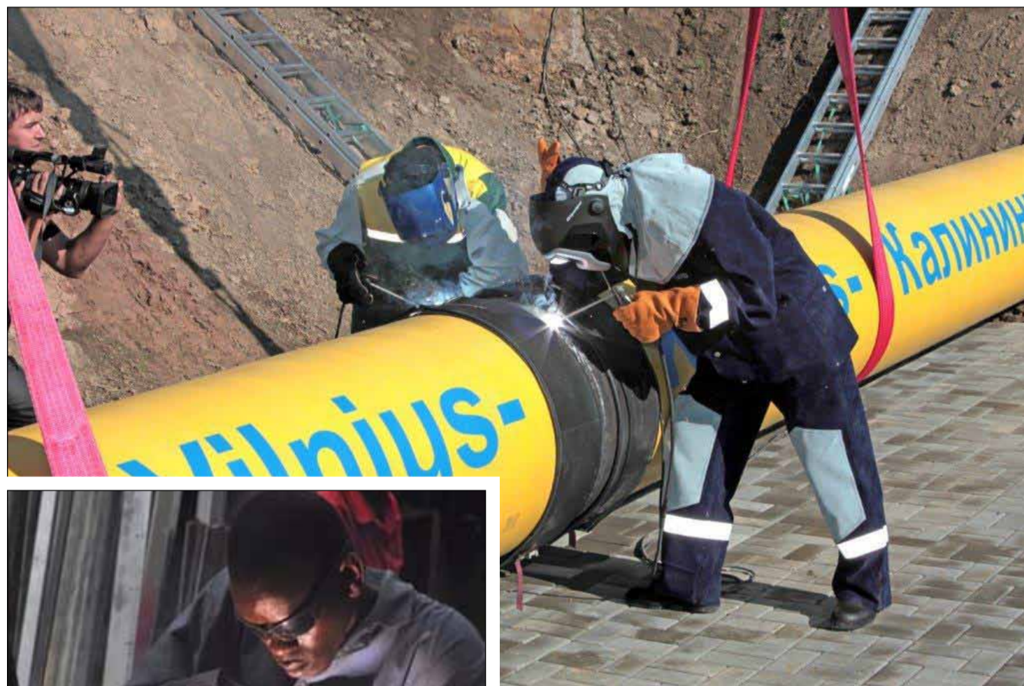
Above: welding a gas pipeline joint in Lithuania.
