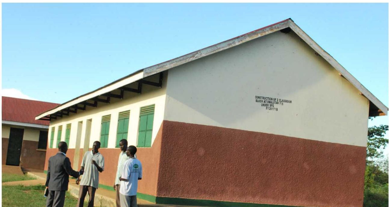
A two classroom block that was constructed at Omalutan Primary School.
