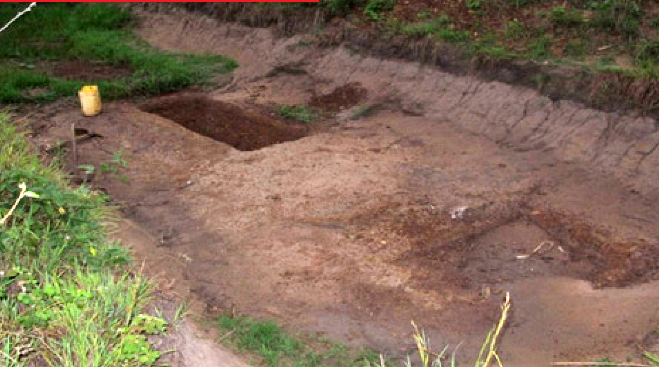
A community built dam for fish keeping and water for animals.
