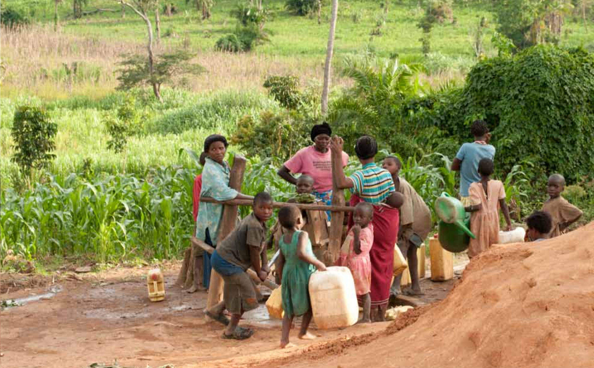
Even the uncooperative zone got a borehole
