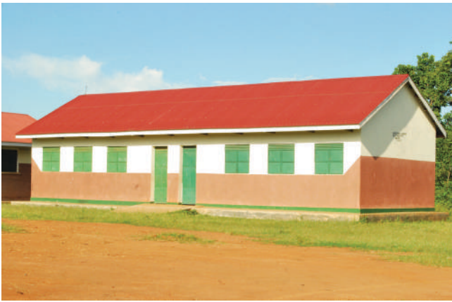
New classroom block constructed in Omulatu Primary School with lobbying efforts by ActionAid
