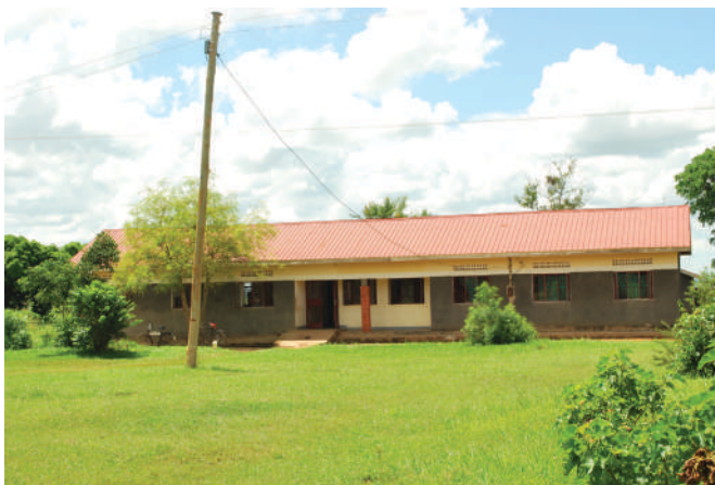
Apopong Health centre III supported by ActionAid to get electricity
